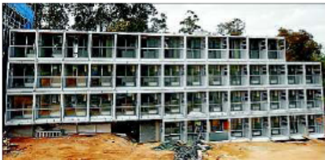
Lego land ... 70 shipping containers become campus accommodation.
